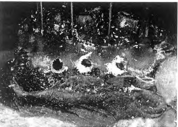
FIGURE 7 Modified access holes are drilled on the side of the "tube template".
